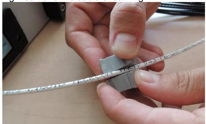
8. Put the inserts into the frame and blind unused holes. Caution: When putting the insert into the frame, the top surface must be smooth.
