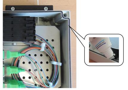
20. Place the cable reserves in the rings on the plastic bottom and secure them with rubber rings.
